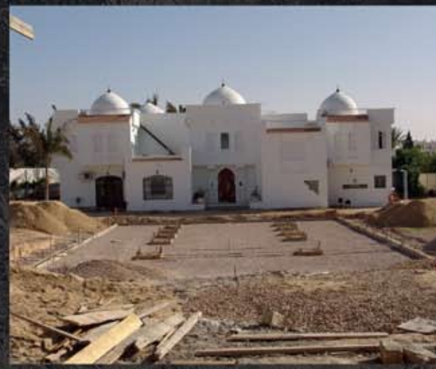
The villa under construction
