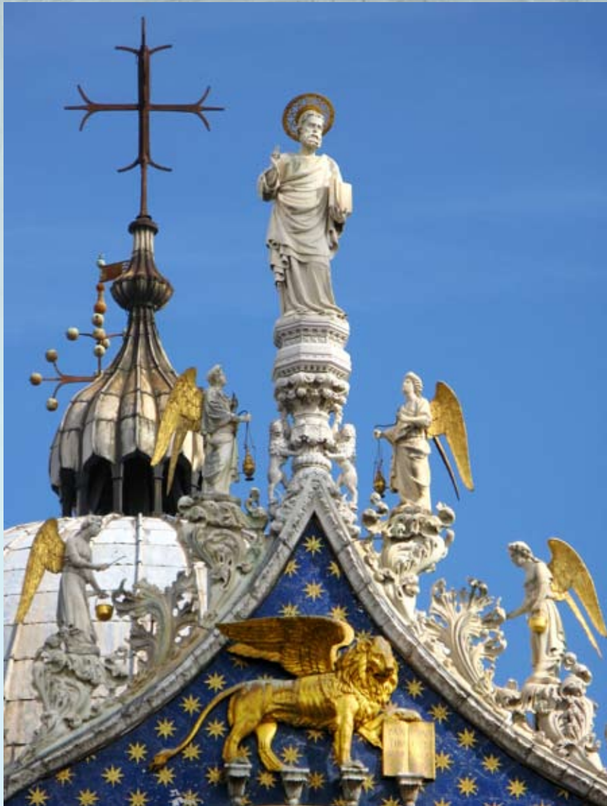
Fig. 3.11 Detail of the rooftop of Saint Mark's Cathedral in Venice
