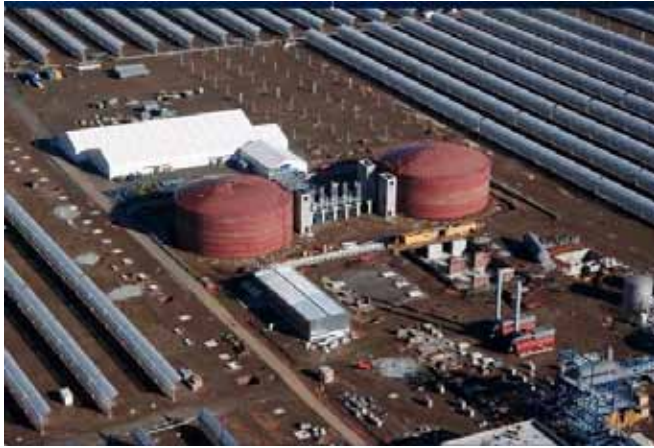
Figure 2 Andasol 1 in Spain - a 50 MW CSP power station with thermal storage for 7 hours full load operation after sunset (Source: Solarmillennium)
