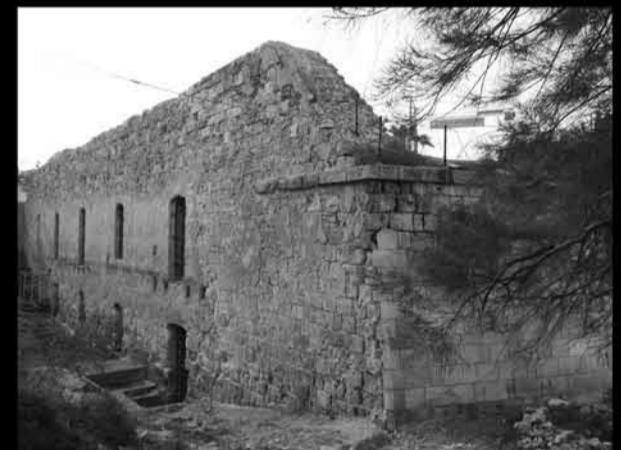
A remaining wall of Nahaseen Fort.
