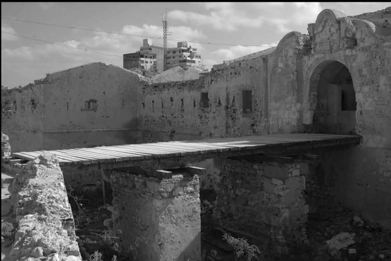
The outer walls, ditch and wooden bridge leading to the entrance of Koussa Pasha Fort. A row of gunholes or slits is visible along the walls.
