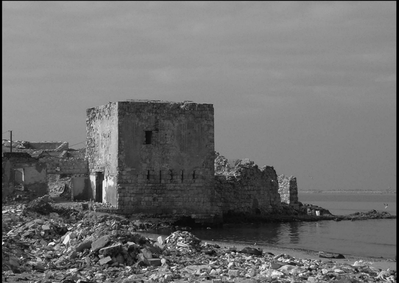
The remains of El Dekhela Fort situated on the shore to the west of Alexandria. A row of gunholes or slits is clearly visible.
