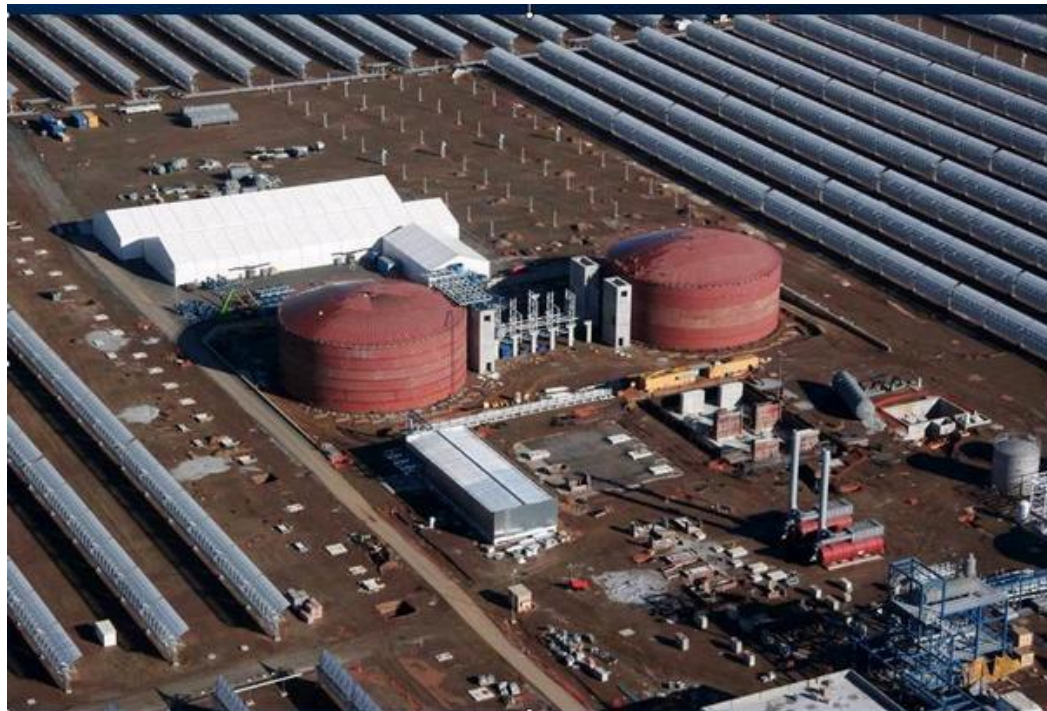
Andasol: 3 x 50 MW 7.5 h storage, Spain
