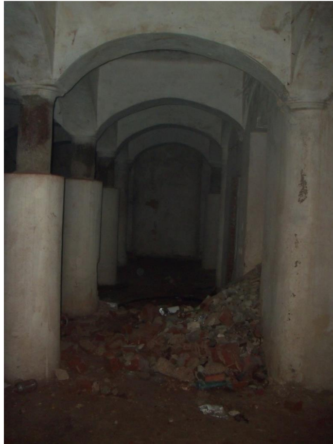
Figure II-12: A photo of the cistern displaying the damage caused by a newly constructed building (Source: the researchers)
