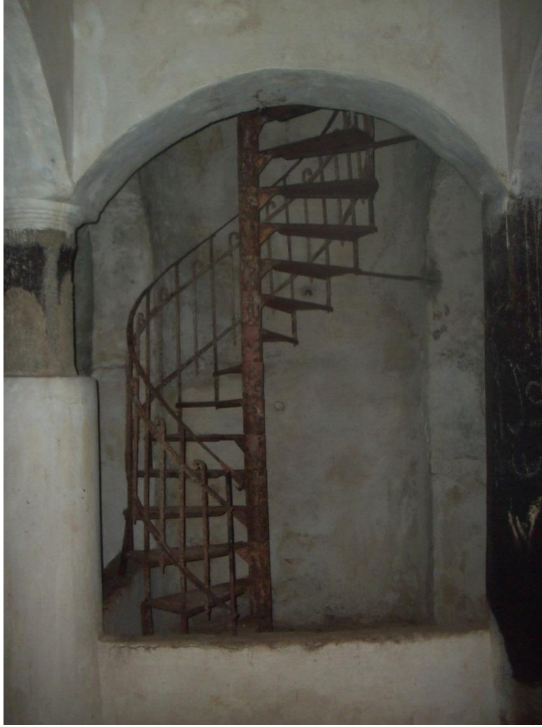
Figure II-11: A photo of the iron spiral stair (Source: the researchers)
