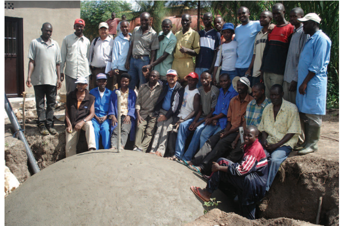
First biogas plant constructed in Rwanda
