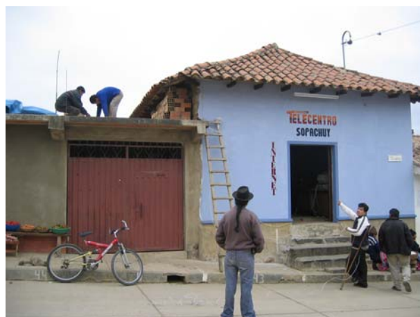
ACLO, watching the progress at the telecentre
