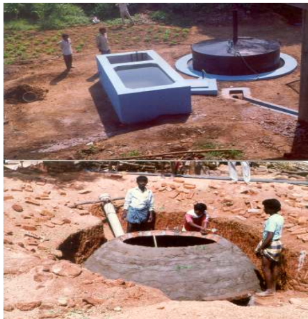
Biogas Plant Models Top: Floating drum Bottom: Fixed dome
