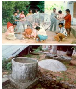
Ferro-cement fixed dome model (in situ construction)
