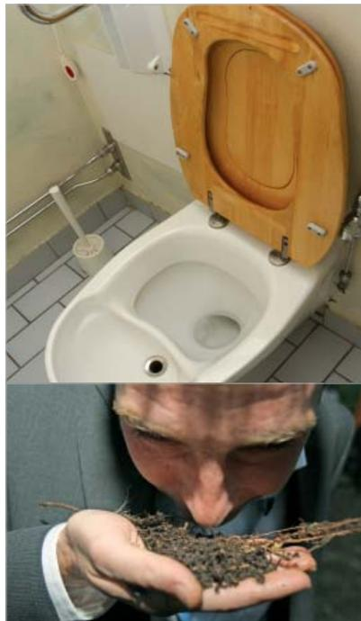
*The double flushing urine diverting toilet Dubletten at Understenshöjden. This model has largely been replaced with the more modern Gustafsberg toilet.*
