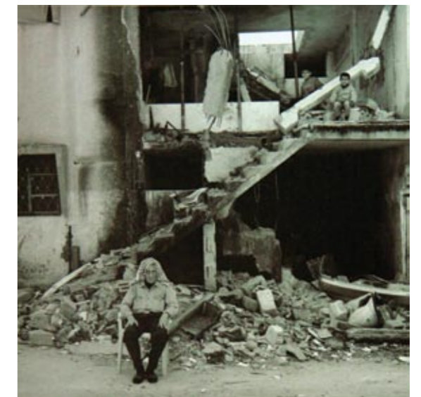
Hussein al-Lawaisi (Abu Khaled) in front of his house in the refugee camp, West Bank, Occupied Palestine. The house has just been demolished by the Israeli Army.
