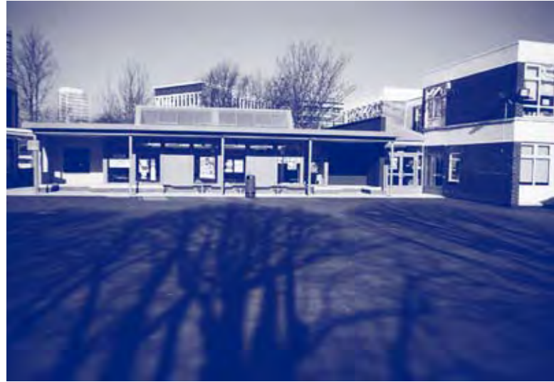
External view of the learning resource centre with alcove seating
