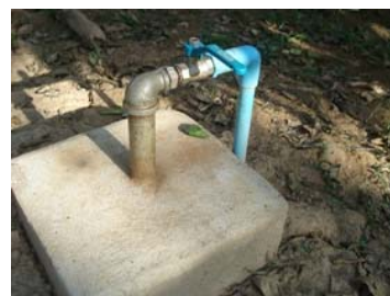
Photo-4.2: Main Gas Pipe & Turret
