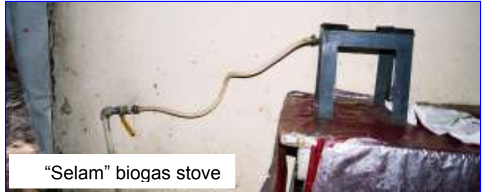
Locally manufactured biogas stove
