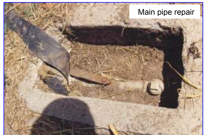
Unblocking inlet pipe
