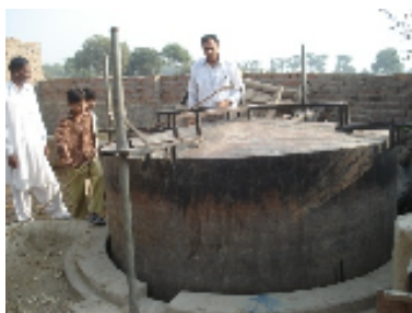
Photo 1: Floating Drum Plant
