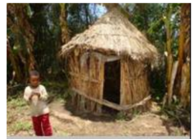
Figure 2. Latrine made from local materials
