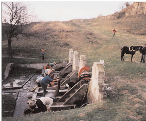
A drinking water well in Garla Mare. The crumbled protection around the well and the lack of cover increase the change of microbiological pollution.
