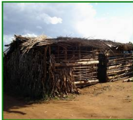
Figure 03: Warehouse in Chimoio (38mm market)
