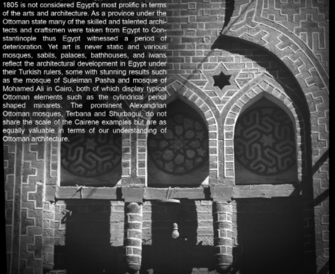
The black and red brickwork, typical of the Delta region, at the entrance to Terbana Mosque
