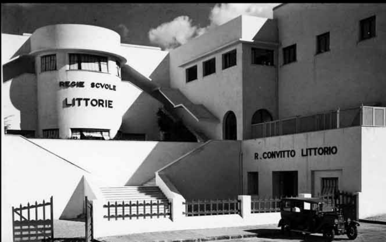
The Littorio Italian School, dates back to 1930. Today it houses part of the Faculty of Agriculture of the University of Alexandria. Photo courtesy of Mohamed Awad.
